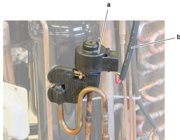
a Expansion valve motor b Expansion valve motor harness
